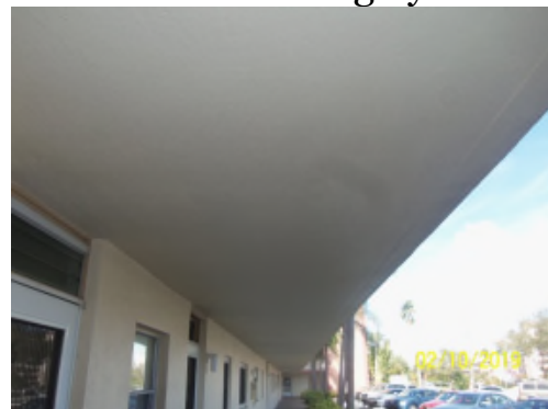
Concrete Roof Deck
